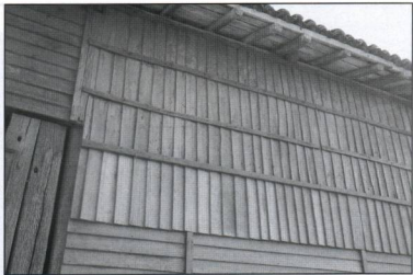
Tavillonnage vertical - Radonvilliers (10)
